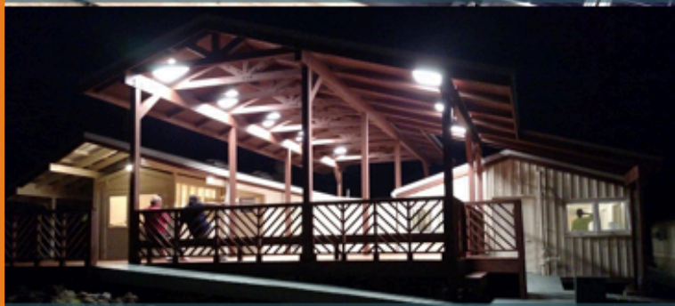
Final PV powered hut.
